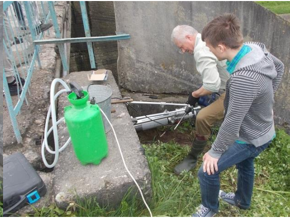
Figure 2. Cores' drilling process and device specification
