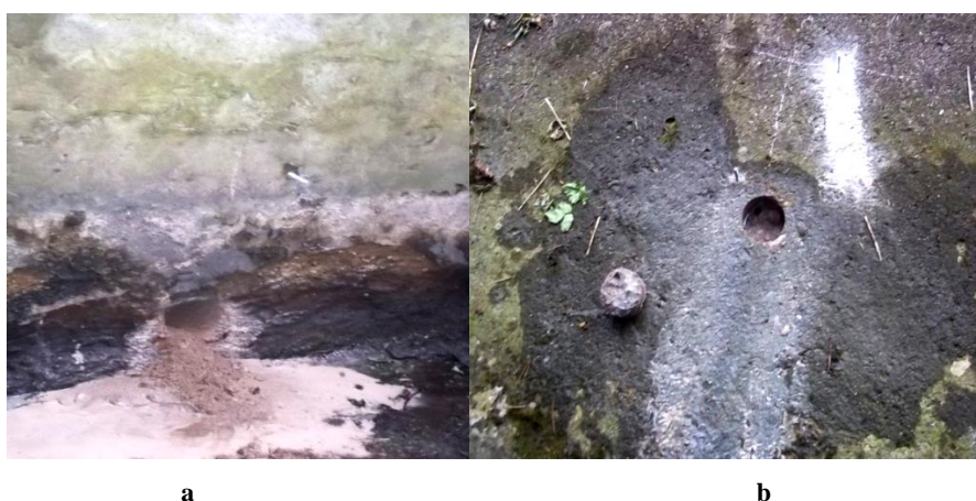
Figure 8. Failed extractions of cores when a) the strength of concrete was too low; b) the thickness of slab was too low
