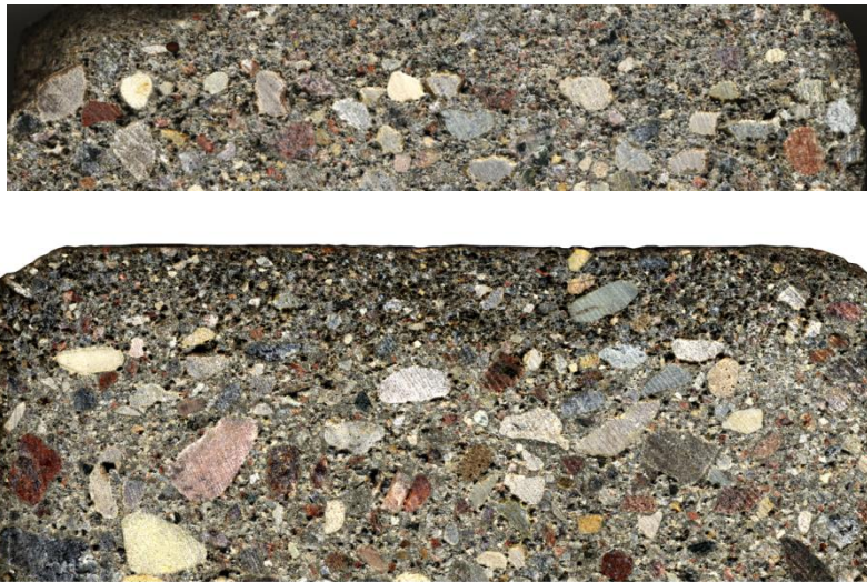
Figure 2. Upper layer of concrete paving block was produced from other fine-graded concrete composition
