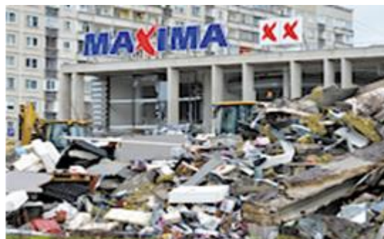
Figure 2. FLAWED: Inspections of buildings in Riga are exposing numerous problems (Lawsuit..., 2013)
